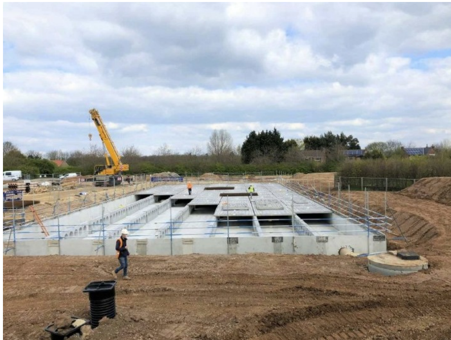
Figure 3.7 Attenuation TC tanks – typical installation (Carlow tanks)
