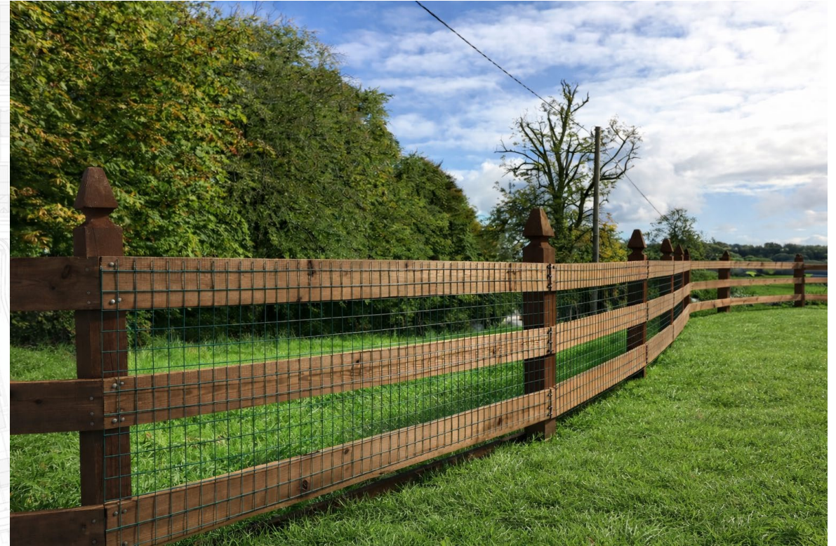
Mesh and timber rail fencing with planting to the inner side
