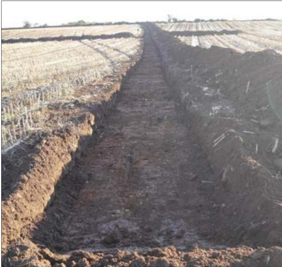
Plate 18: View of the excavated Trench 14, facing south-southeast
