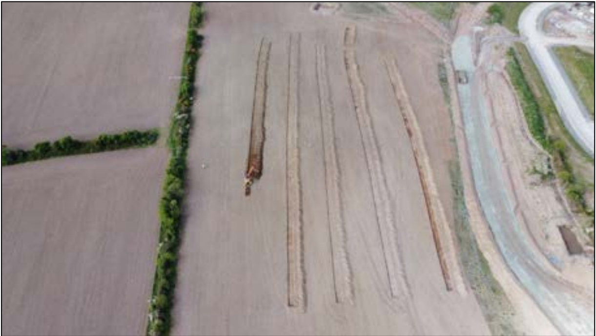
Plate 1: Aerial view of trenching works within western land parcel, facing west
