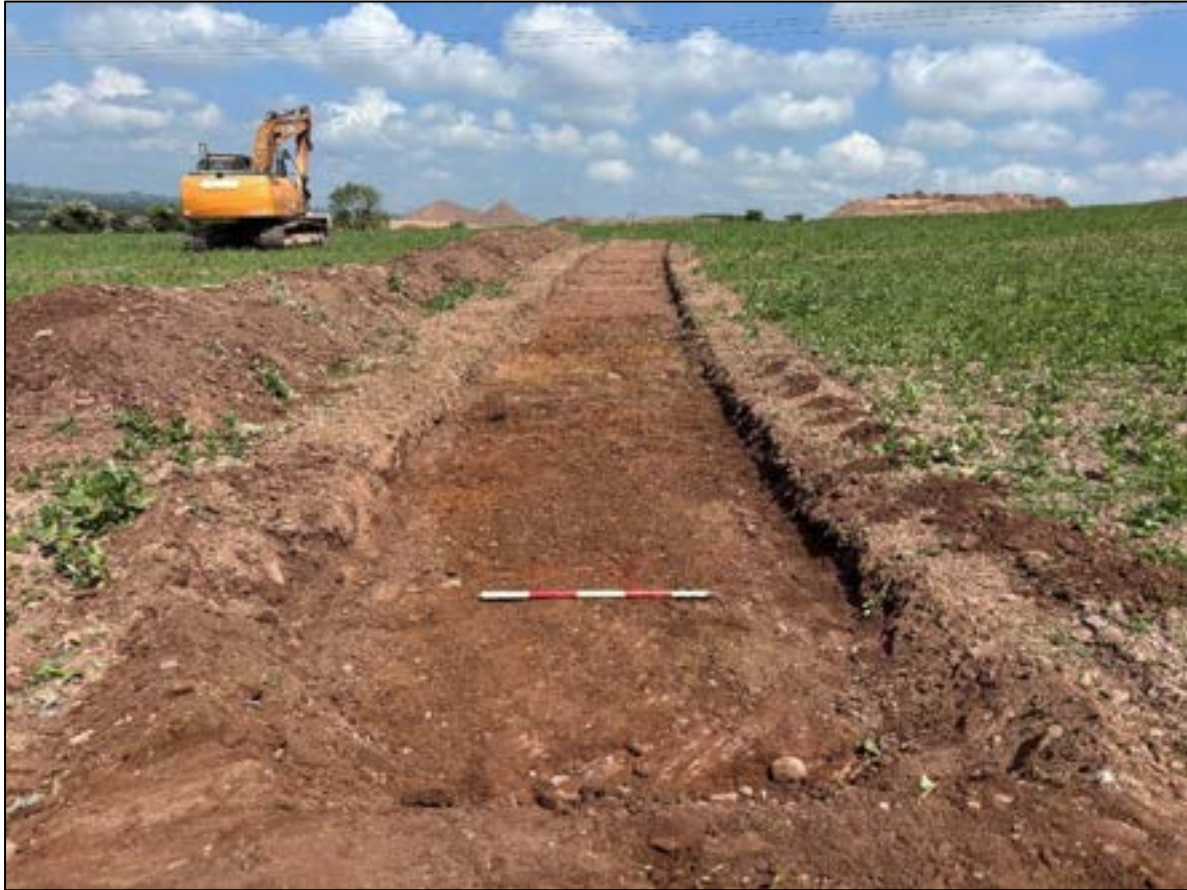
Plate 25: View of portion of Trench 10 south of overhead powerlines looking north
