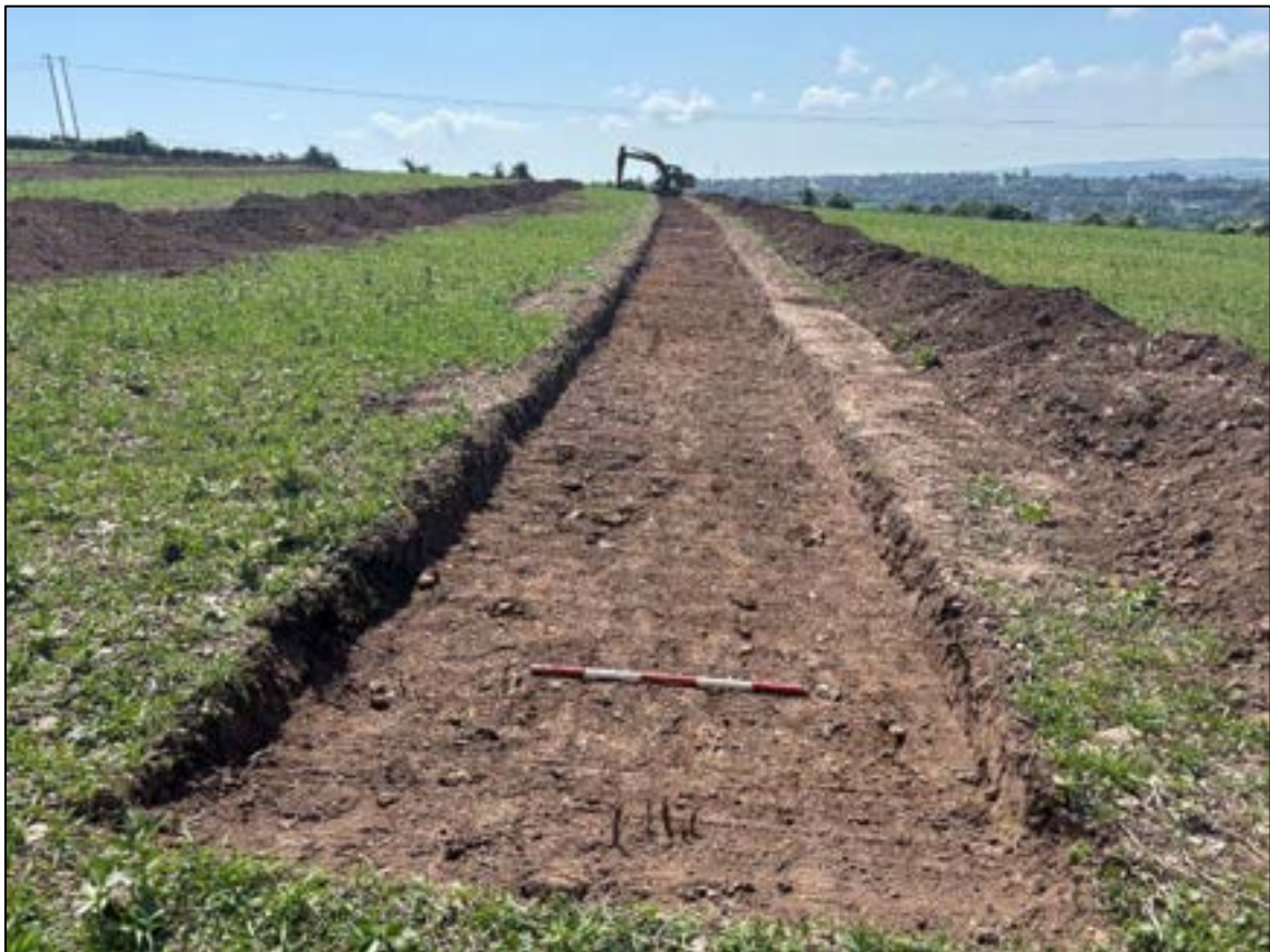
Plate 30: View across the completed Trench 12, facing south
